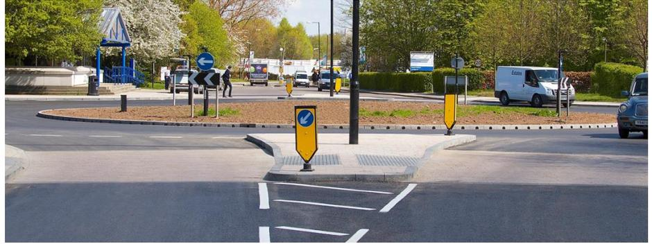
We were appointed by Warwick University to upgrade one of the main entrances into campus. Works included extensive service alterations, creation of four granite crossings, narrowing island approach lanes to increase pedestrian safety, construction of two new bus lay-bys and resurfacing of roads and footpaths.
